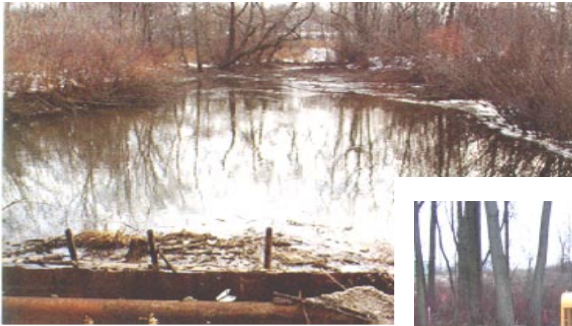
ABOVE: Contaminated sediments & scum temporarily captured behind the failed, in-stream dam at Lakeside.
